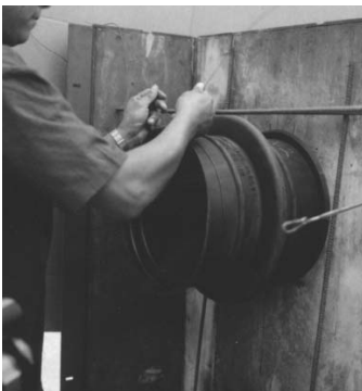
5. For additional stability, it's necessary to secure the sleeve with wire to the rebar. Inset the other end cap firmly and check that second end cap is positioned correctly and close the form.
